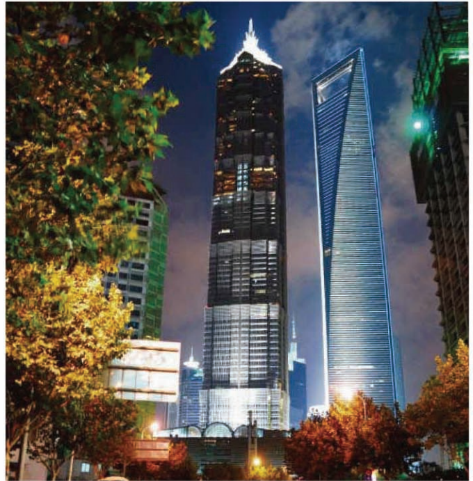
Sites where compact size and light weight are required (Urban multistory buildings, etc.)
