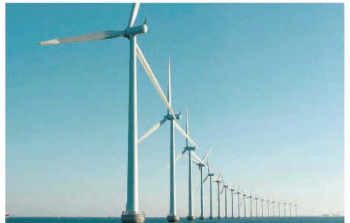
Wind power site
